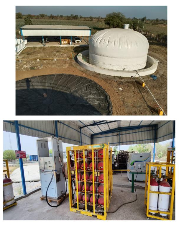
A vehicle's emission with the enriched biogas fuel (Bio-CNG) meets to the BS IV emission norms. There is no significant change in fuel economy of the vehicle fuelled with the enriched biogas (24.11 km/kg) as compared to base CNG (24.38 km/kg). The biogas plant such as the project activity, are significant and growing contributors to achieve world climate-neutrality by 2050.
